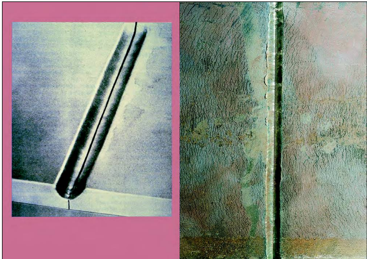
Figure 3.65—Illustration of Joint Preparation Using Mechanized (left) and Manual (right) Air Carbon Arc Cutting
